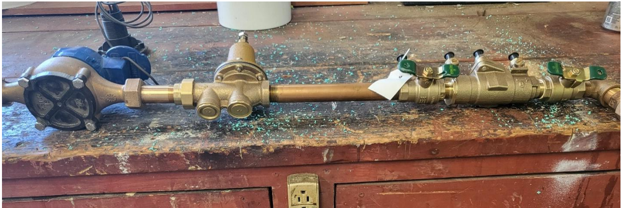
Meter Assembly, with pressure regulator and Backflow Prevention Valve (BFPV). The BFPV is located outside of the city meter box in a separate box.
