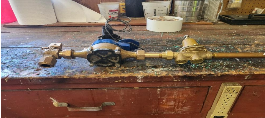
Standard Meter Assembly, with pressure regulator
